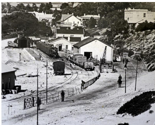
Simon's Town Station in 1905 showing the goods shed. The turntable would have been behind the train in the station.
