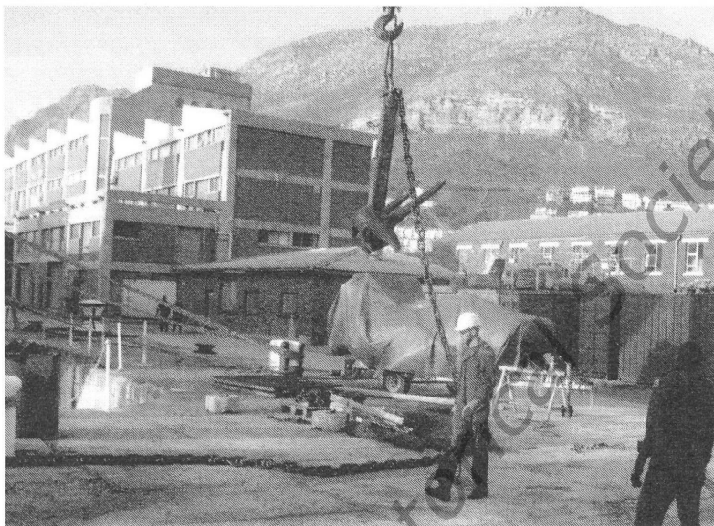
GROUND TACKLE FOR THE CASTOR BUOY SUSPENDED FROM A CRANE HOOK. THIS VIEW SHOWS THE DOCKYARD "AFLOAT TRADES" WORKSHOPS AND THE QUARRY FROM WHICH STONE WAS SENT DOWN TO BUILD THE BASIN WALLS AND ORIGINAL WORKSHOPS. – Photo : Captain Wallace-Bradley.
